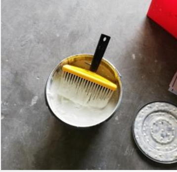
Application of EZY-NET® with block paint brush or airless on surface polluted with sooth (caused by fire).
