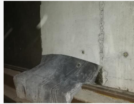
Peeling off EZY-NET® film after it has dried out, resulting in a clean surface.
