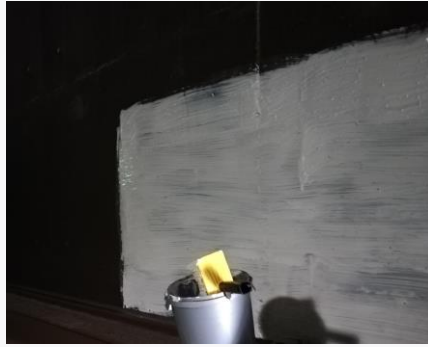
Application of EZY-NET® with block paint brush or airless on surface polluted with sooth (caused by fire).
