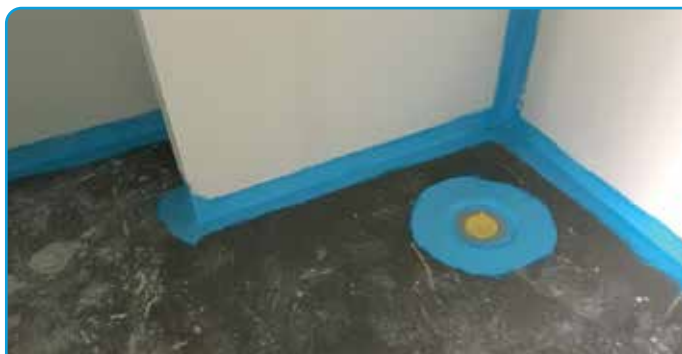
INSTALLATION OF PRIMER 43 + SANIPROOF BRUSH IN CORNERS AND AROUND GULLIES
