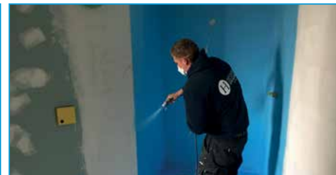
SPRAYED WITH SANIPROOF LIQUID IN 2 LAYERS
