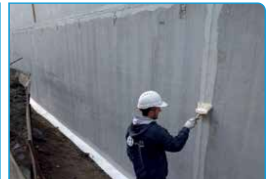
WATERPROOFING OF BASEMENT JOINTS
