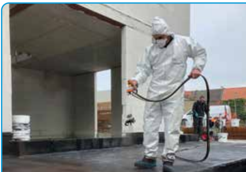
WATERPROOFING OF BURIED STRUCTURES
