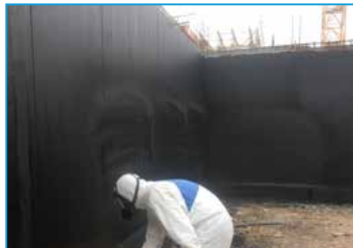
WATERPROOFING OF UNDERGROUND WALLS
