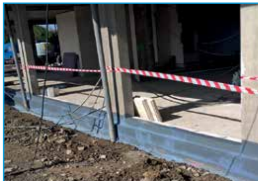
WATERPROOFING OF FOUNDATION FOOTINGS
